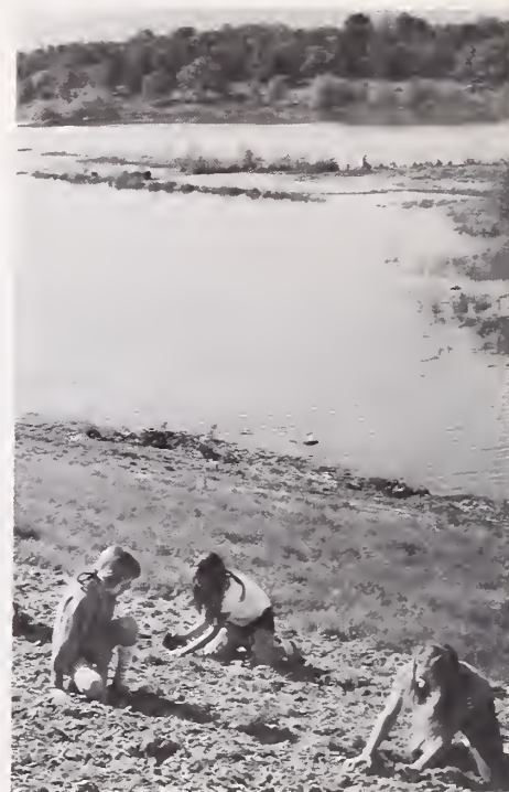
Girl Scouts plant and mulch the slope of a small dam to help keep the soil from washing into the reservoir and polluting the water.
